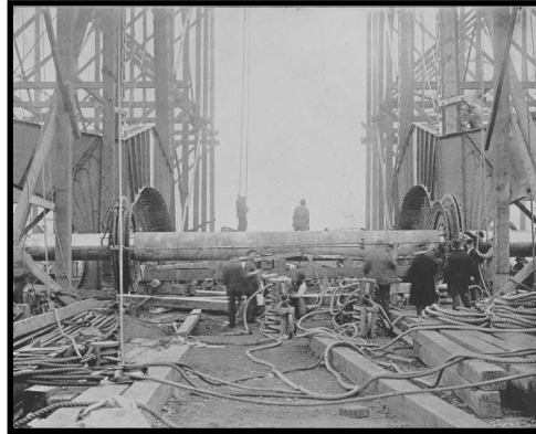
The 70-ton axle of the Ferris wheel after its arrival in Chicago in 1893.
